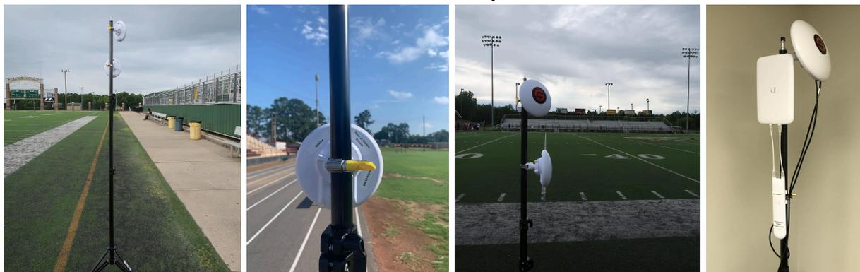
\*station should be placed at the 35 yd line, farthest from the bleachers with a clear line of sight to the press box antenna
